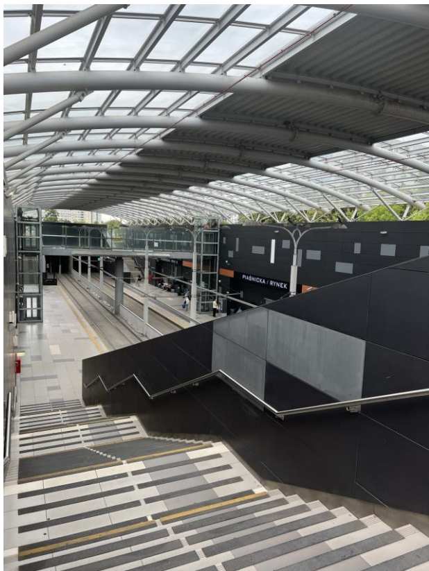
Fig. 2. Interior view of the Piaśnicka/Rynek tram stop
