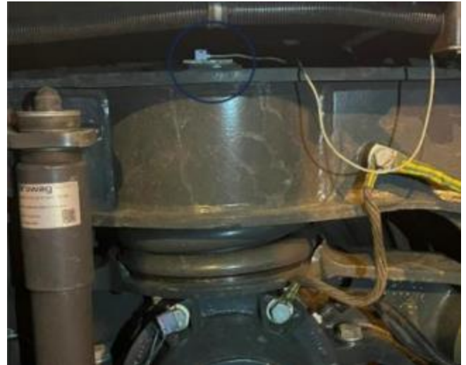
Fig. 9. Measurement point 1 localized on the train bogie
